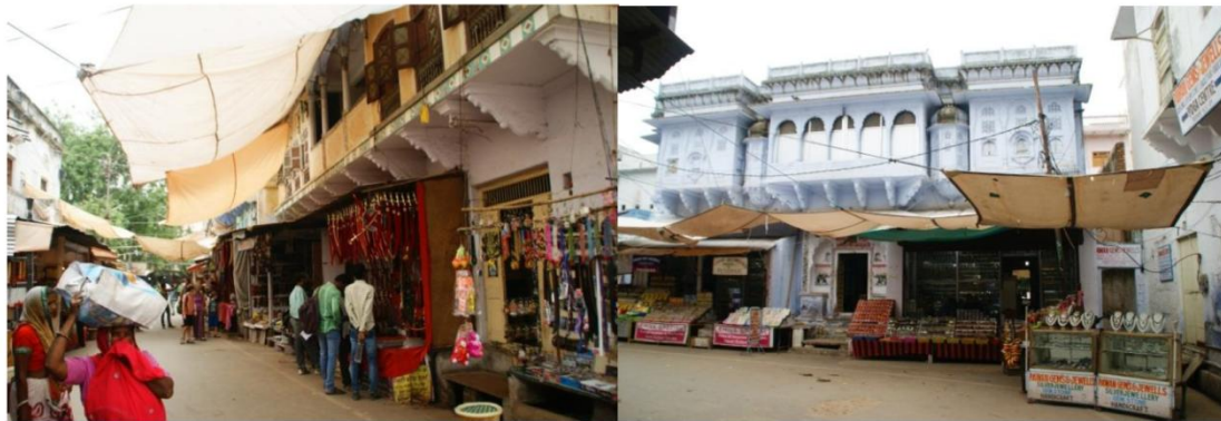
Cloth covering over the streets disturbing the elevation of historic facades.
